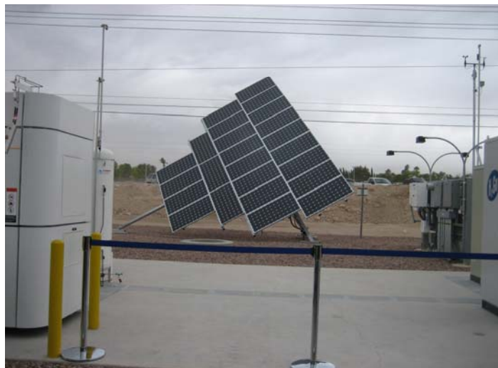
Solar panels collect energy from the sun to create hydrogen for fueling vehicles at the Las Vegas Valley Water District.
